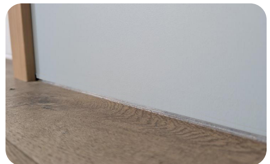
enhanced behavioral health base detail with scribed cladding and security-grade caulking.
